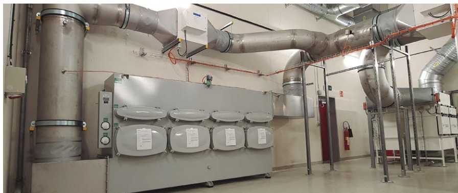
Nuclear filters - CERN AD TARGET
