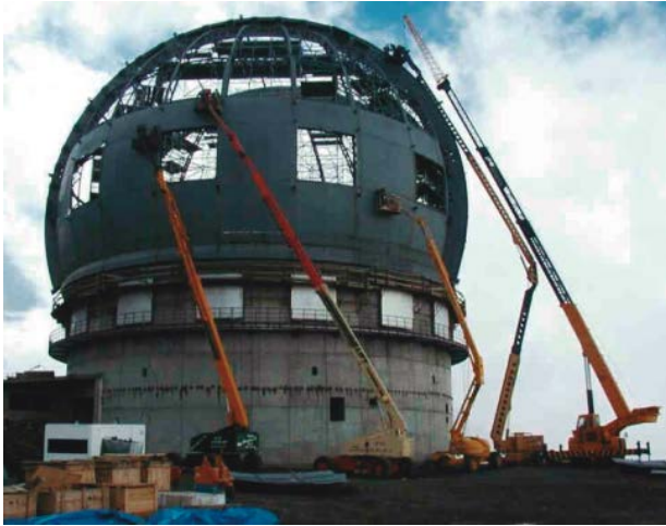
GRANTECAN dome erection
