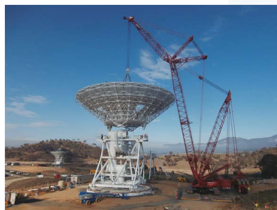
DSN 34m antenna installation in Australia
