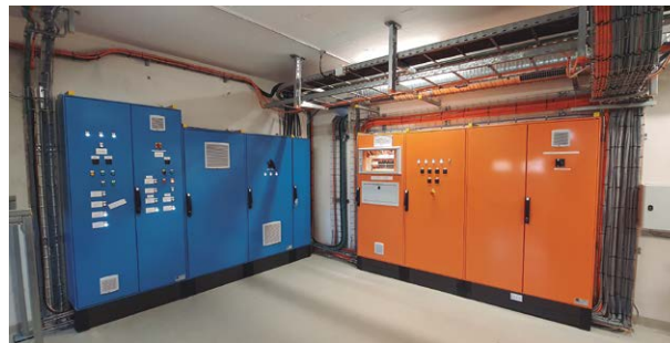
Electric cubicles - CERN AD TARGET
