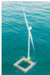
Demonstration of advanced floating offshore wind generation ➢ Water depth is form 50m to100m ➢ Weight reduction of floating Offshore wind turbine system To achieve cost reduction
