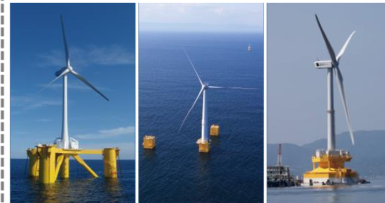
Fukushima floating offshore wind farm demonstration project from left, 2MW compact semi-sub, 7MW V-shape semi-sub and 5MW advanced spar
