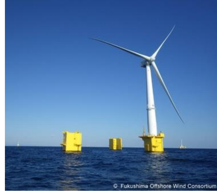
2 nd 7MW turbine (Mitsubishi hydraulic type) on semi-sub type floater (Mitsubishi) , under commissioning now
