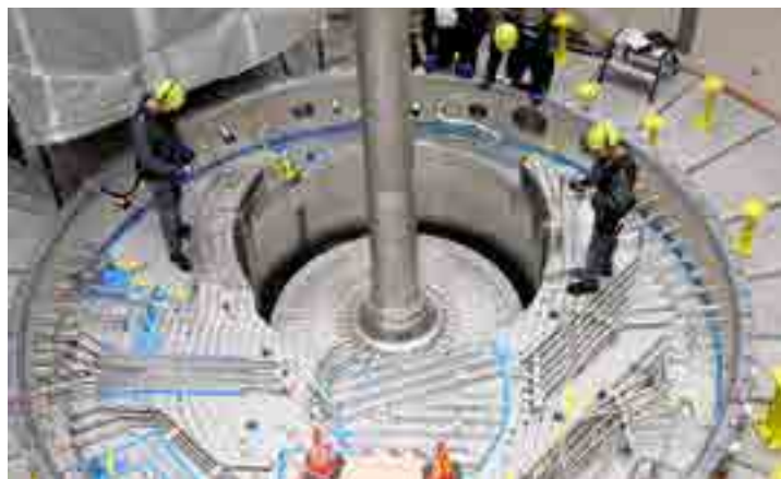
Target Wheel installation at ESS. Image courtesy of ESS
