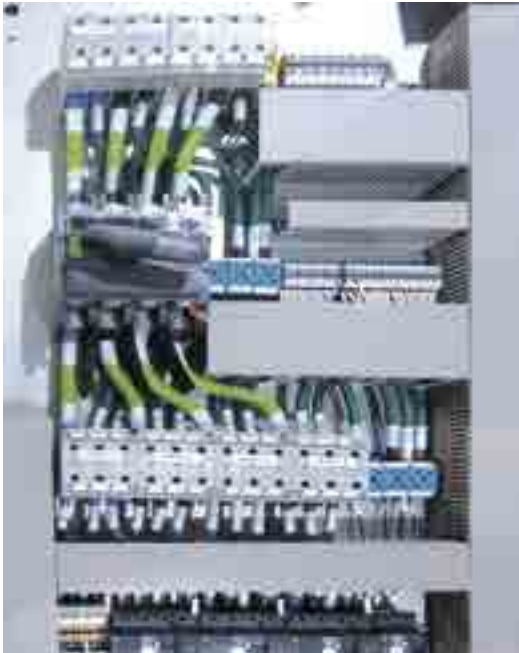
Upper part of the HSB01 distribution board including high current distribution devices
