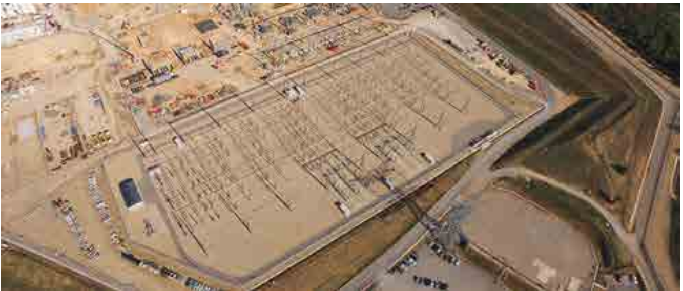
The very high voltage electrical substation on the south side of the platform (Photo I0 EJF Richie)
